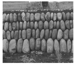
Even when the clawdd is built with "flat-layed" stone, rather than pitched, it is not simply a dry stone wall with an earth infill. Cloddiau are considerably wider than dry stone walls to enable adequate compaction of the core. In addition the
